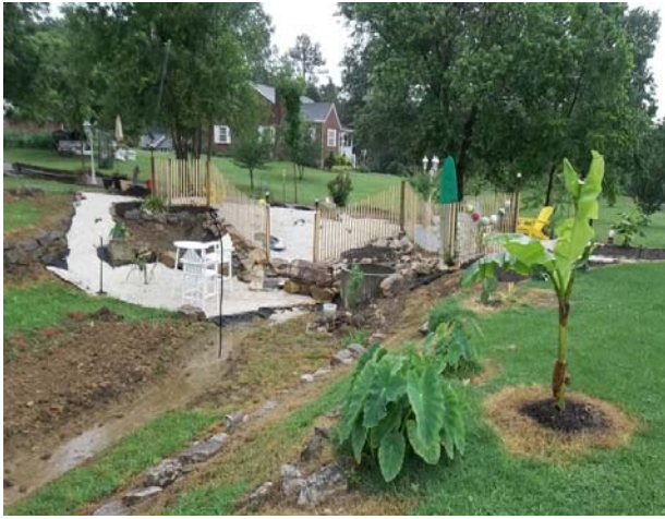
Detention pond turned beach! Placing objects in a detention pond will cause damage to the objects as well as contribute to localized flooding.
