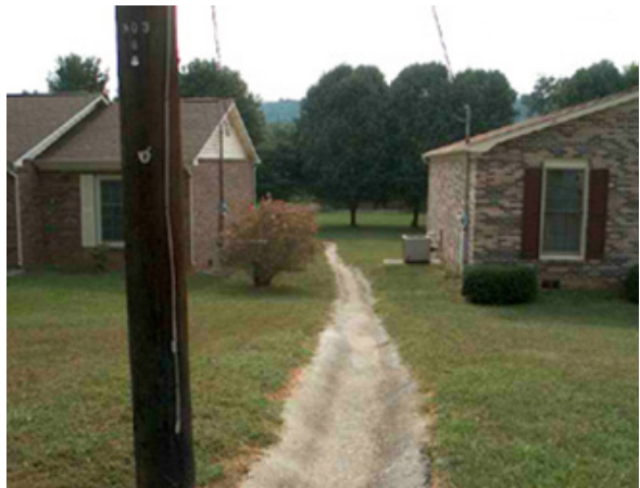
Example of a concrete-lined ditch
